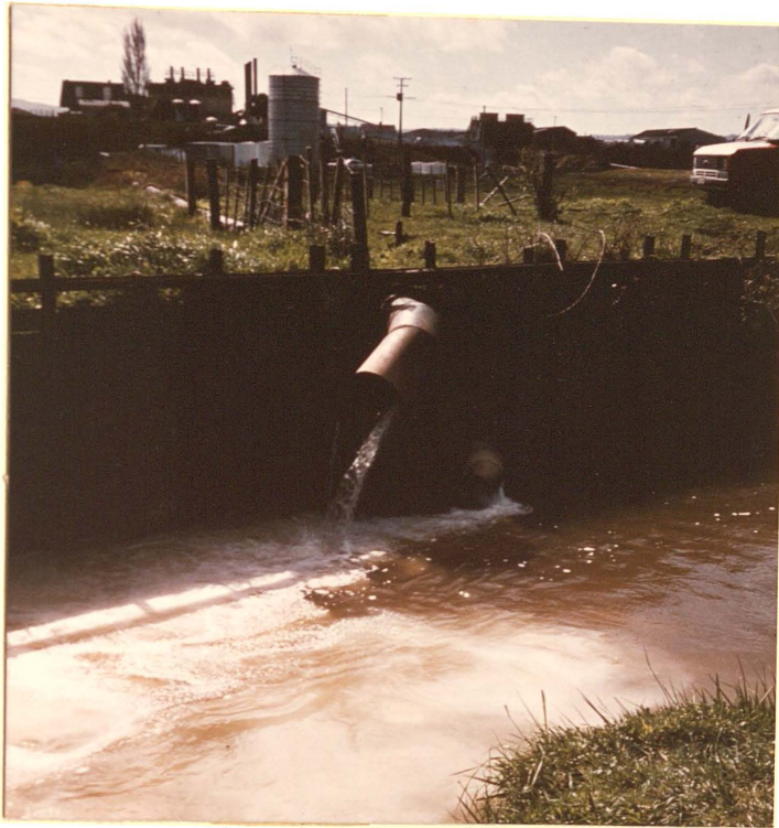
Plate 3.4 Waharoa dairy factory effluent discharge to the Waitoa River.
