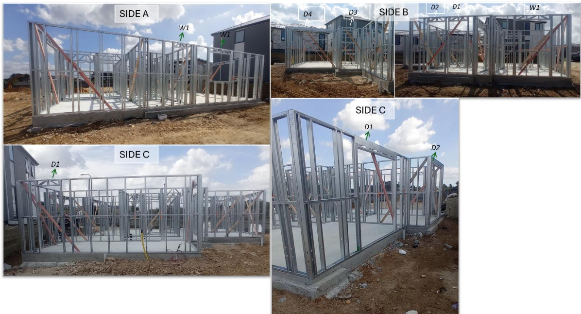
Fig. 14. Exterior faces of the Site 1 structure, labelled A–D, with detected door openings (D) and window openings (W) annotated by instance.
