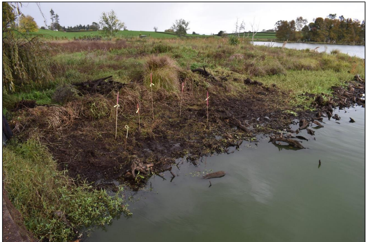
Figure 7.1.4. The northern end of Area A cleared of vegetation.
