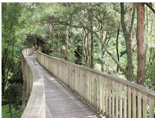
Figure 8: A wooden walkway, A.H. Reed Memorial Park, New Zealand Source: Whangarei District Council (2016), Used with permission
