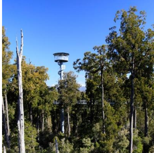
Figure 12: An observation tower, Westcoast: tree top walk and cafe, New Zealand Source: West Coast: Tree Top Walk and Cafe (2017), Used with permission
