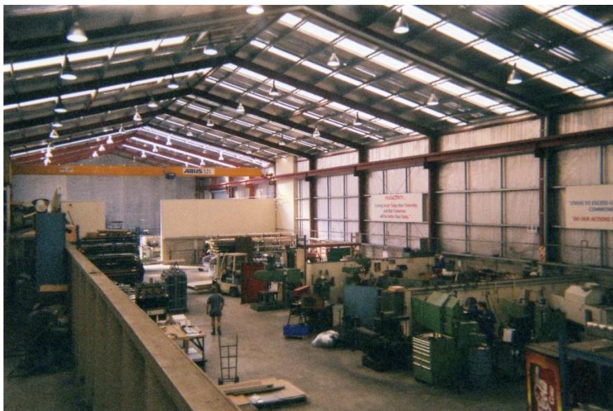
Plate 25: The Stafford shop floor.
