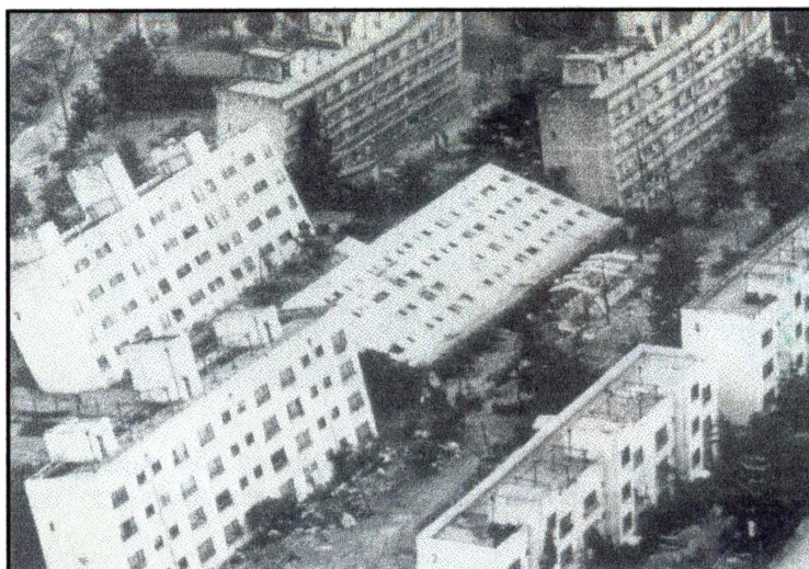
Photograph 12: Earthquake damage. A photograph provided for "stimulated recall" during student interviews (Press and Siever, 1994, figure 18.19)
