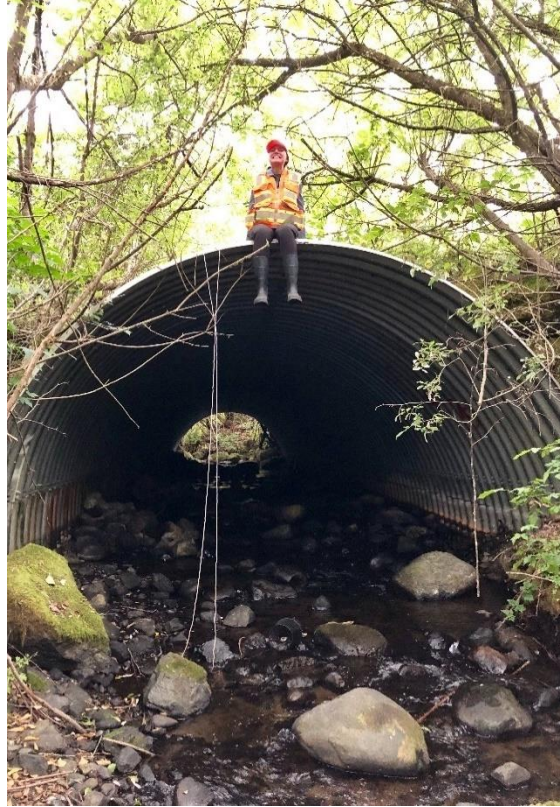
Arch culvert, King County, Washington, USA
