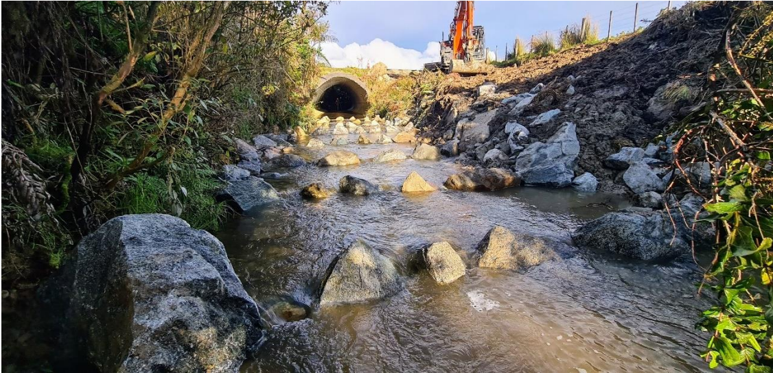
Construction of rock ramp on Mill Creek, Greymouth, New Zealand
