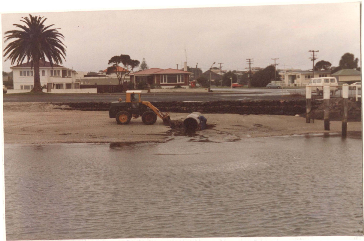
Plate 7.2 - Southeastern end of Pilot Bay beach on 15 August 1984 showing stormwater discharge eroding the beach and remedial work underway to prevent further collapse of the extended outfall.
