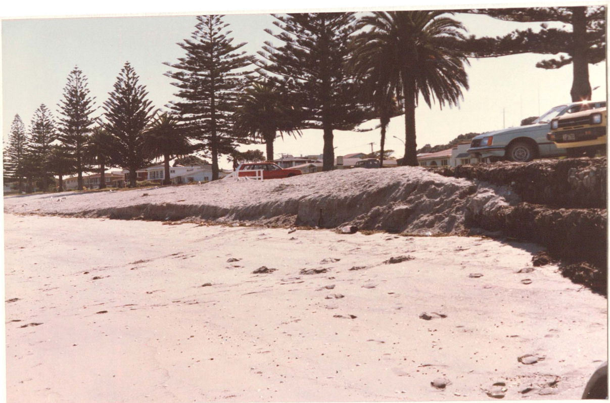
Plate 7.4 - Erosion at the southeastern end of Pilot Bay beach on 13 April 1984, shortly after completion of landscaping of the renourished beach.
