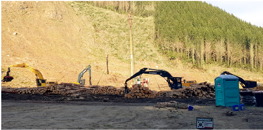
Figure 2.3: Typical cable hauler skid site
