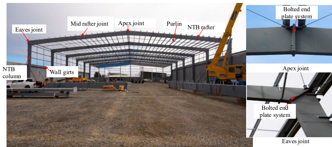
Figure 1-1 Photograph of cold -formed steel NTB portal framing system and its joints (Donovan Group Ltd.)
