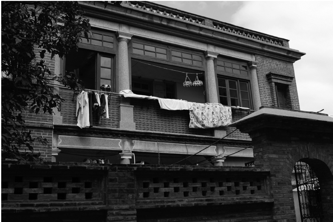
Plate 13: Building with Tuscan columns
