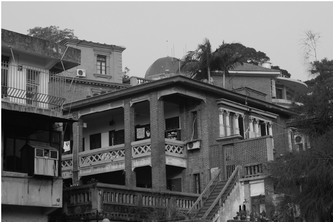
Plate 22: Building with Corinthian columns and French colonial windows
