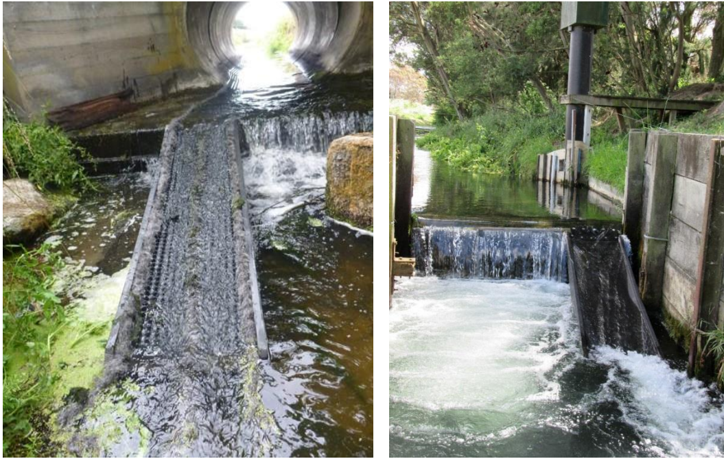
Figure 4.2: Ramp installations in the Awanui Stream (left) and Irongate Stream (right).
