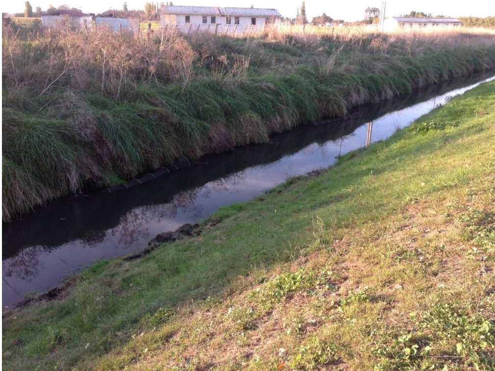
Figure 2.3: Awanui Stream, upstream of culvert. Note: Reaches downstream of bridge have more natural channel form and sinuosity.
