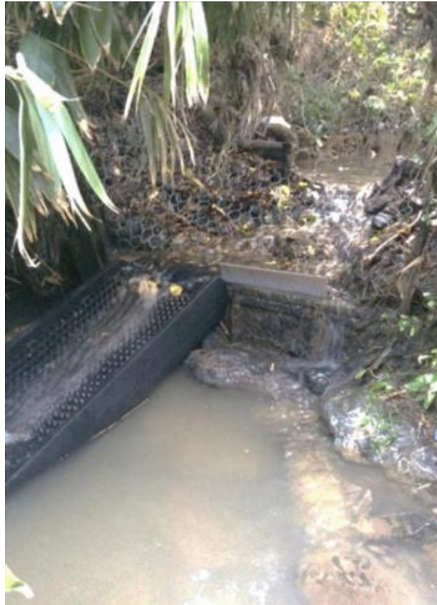
Figure 5.3: Flexible baffles (ATS Environmental) directing water over a floating fish ramp in Nelson. Photo credit: Tim Olley, Fish and Wildlife Services.
