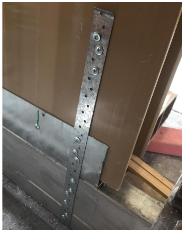
(d) 25mm steel strap fixing (right)
