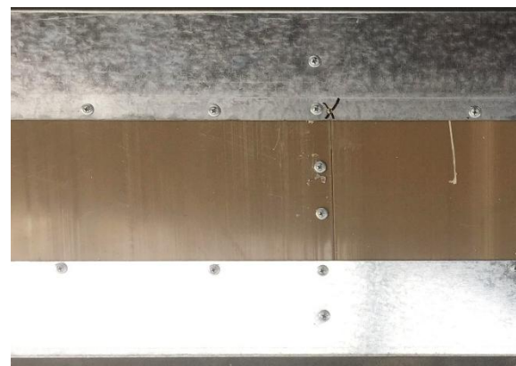
(b) Lintel fixing details
