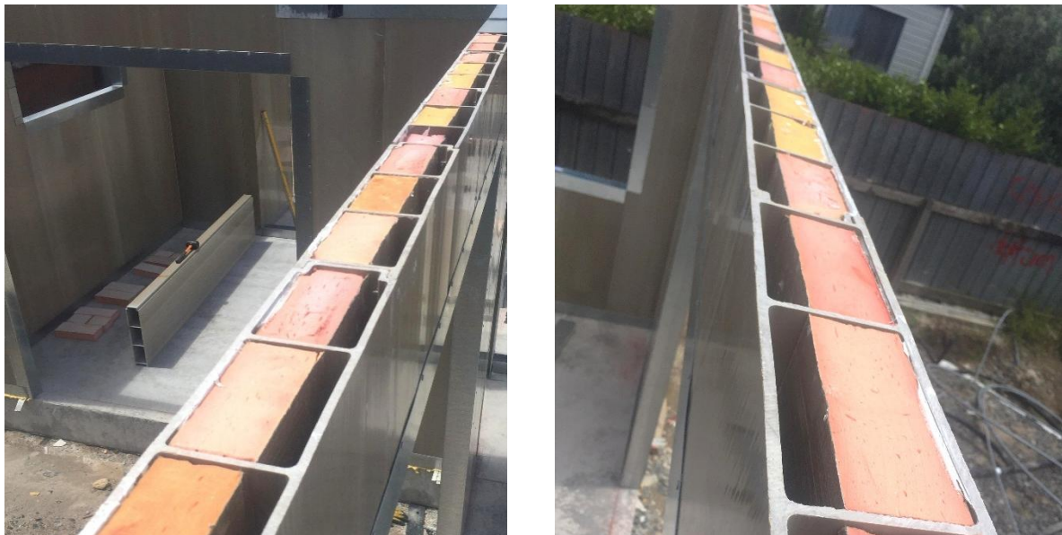
Figure 50-FRP wall panel system lintel insulation detail
