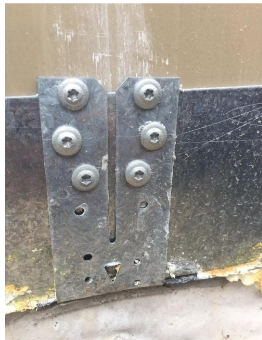
(b) Bracing plate in the panel walls
