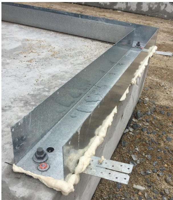
(a) Bracing plate fixed into the foundation
