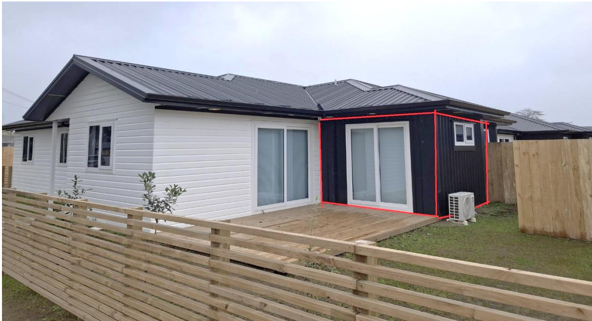
Figure 67-The Investigated master bedroom (circled) of the case study building
