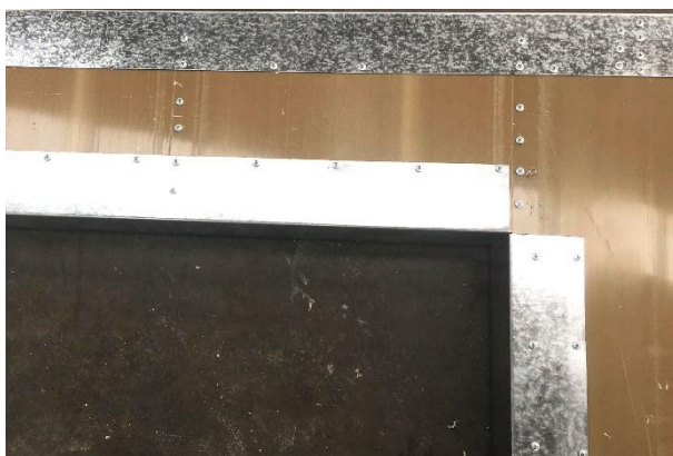
(a) Lintel and wall panel connection
