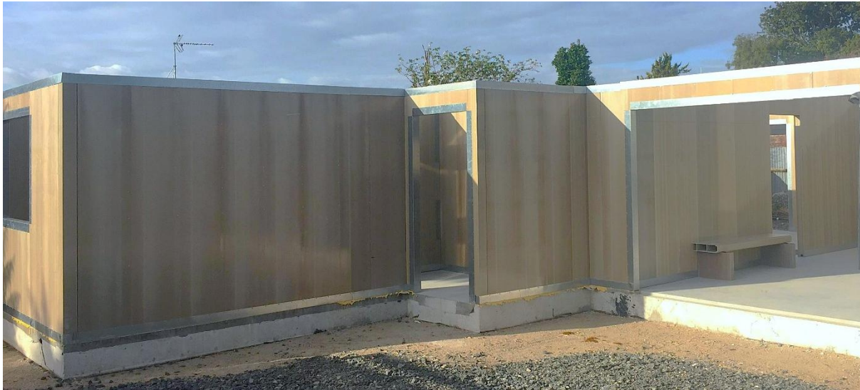
Figure 49-Installation of lintels in the case study building with an FRP wall panel system
