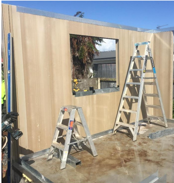
a) FRP panel walls (internal view)
