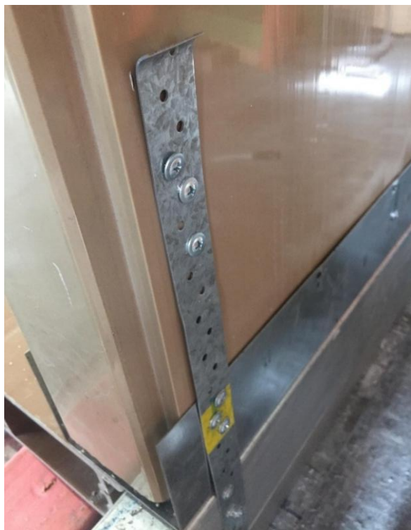
(c) 25mm steel strap fixing (Left)
