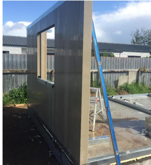
b) FRP panel walls (corner view)
