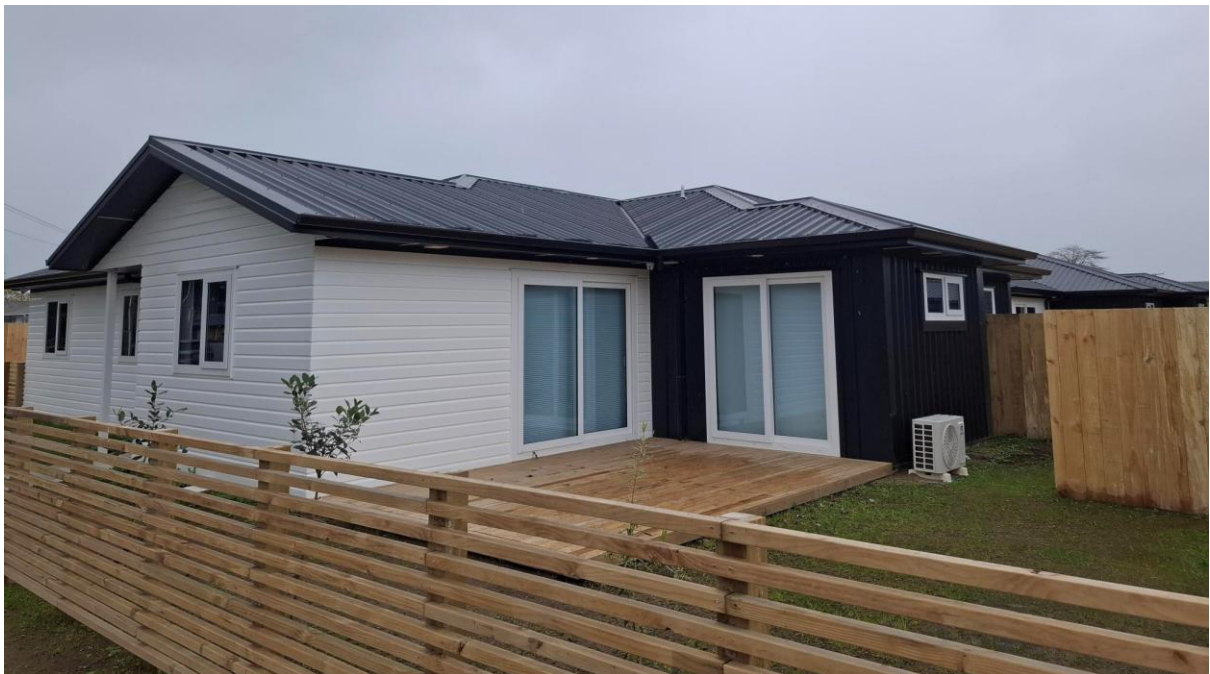
Figure 4-The completed duplexes built with FRP wall panel system (back view)
