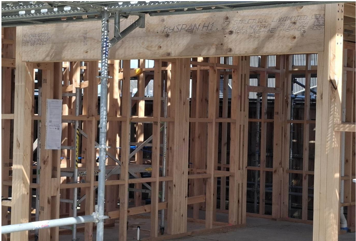
Figure 46-Conventional solid timber lintel in time framing structure
