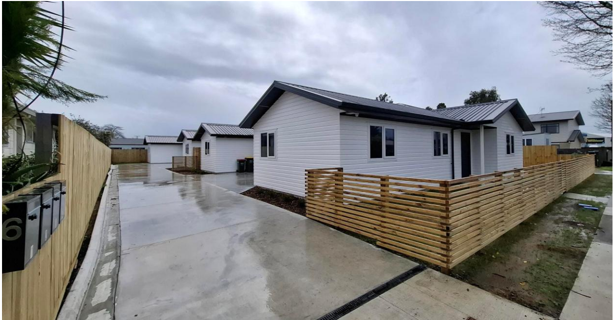
Figure 3-The completed duplexes built with FRP wall panel system (front view)
