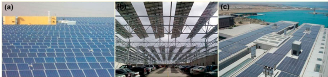
Figure 22: Solar PV projects in KSA: (a) King Abdullah Petroleum Studies and Research Center Solar Park; (b) Saudi Aramco solar car park, and (c) King Abdullah University of Science and Technology Solar Park. (Mas’ud et al., 2018)
