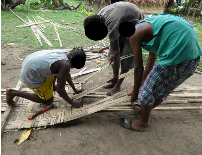
Figure 7: Constructing house wall with flattened bamboo, 2017
