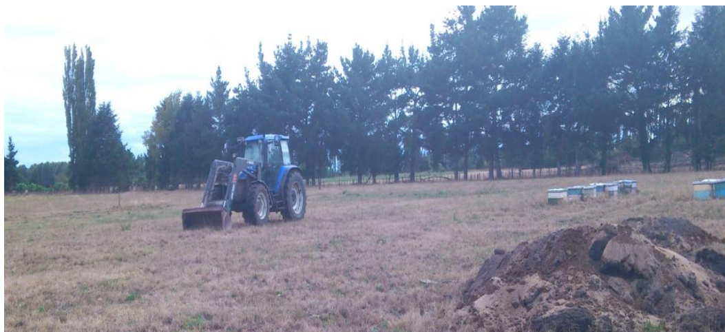
Figure 3.7: A tractor with a bucket loader excavating pits.
