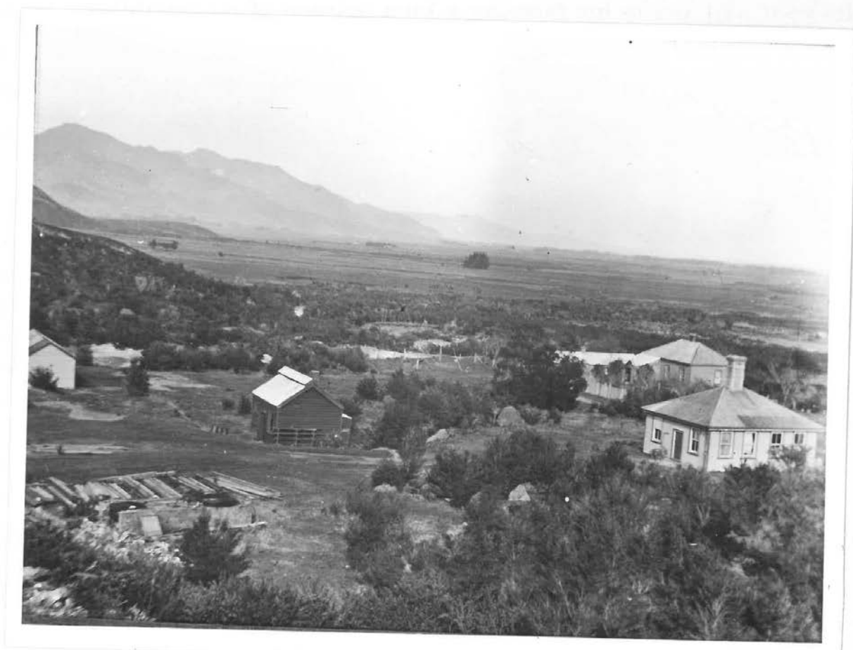
Figure 9: J.S. Hill, assay house and other buildings near Waiorongomai battery, c. 1912, Eric Hill Collection.
