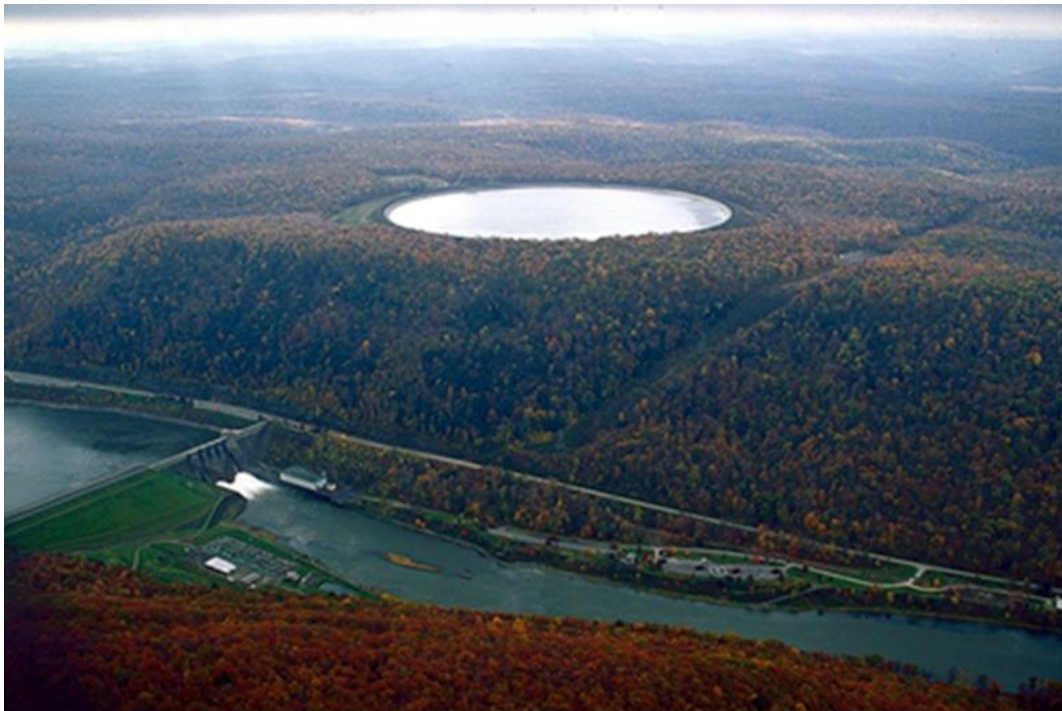
Figure 2.7 Seneca Pumped hydro energy storage constructed in 1970, on Allegheny River, Pennsylvania USA, 435MW.
