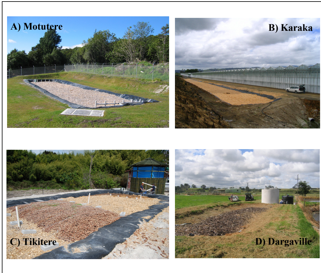
Figure 1.1 Photos of four operation denitrification beds. A) Motutere, (Lake Taupo, NZ) treating municipal effluent nitrified by an SBR plant. B) Karaka, (Auckland, NZ) treating hydroponic glasshouse discharge. C) Tikitere, (Rotorua, NZ) treating nitrogen in a geothermal stream. Note trickling filter in the background for nitrifying the water before flowing into the bed. The carbon substrate is a combination of maize cobs and woodchips. D) Daraville, (NZ) treating dairy shed effluent. Note the MBR plant in the background for nitrifying the effluent.
