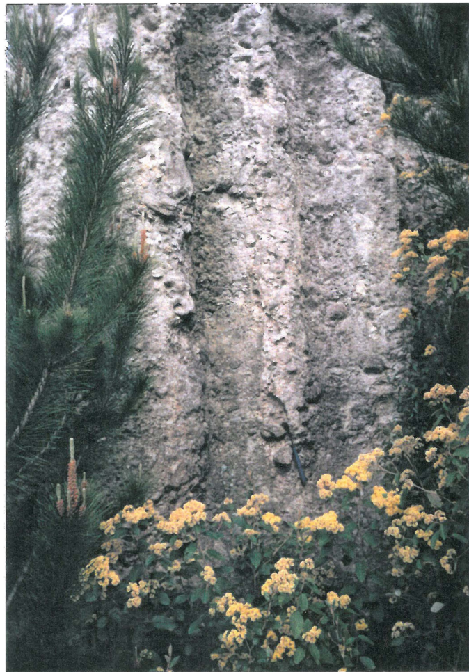
Figure 2.21. Mass emplaced block and ash deposit resulting from instability of the Glassy Dome Rhyolite (unit 2b) exposed in fluted bluffs adjacent to Rangipo Road (T12 649475). Hammer is 33cm long.
