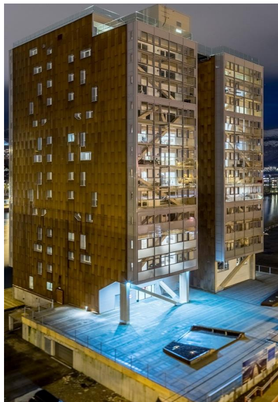
Figure 1 Treet—Timber tower apartment building in Bergen [16].
