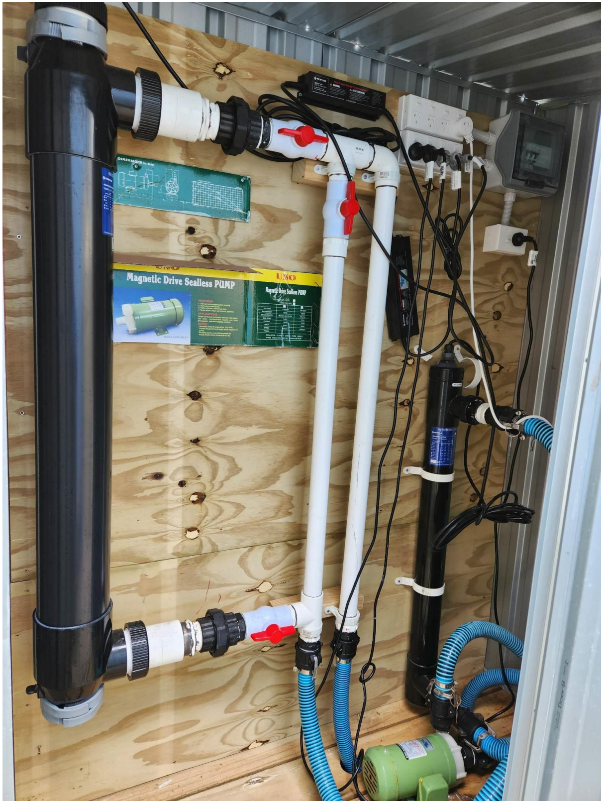
Figure 9b: Photo showing the UV sterilization and pump set up inside an enclosed shed to outside of the laboratory.
