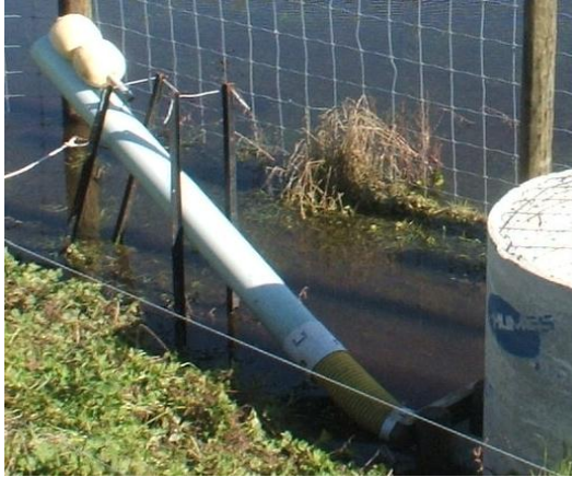
Figure 2.2: Floating decant suspended by a pin to retain 'first flush' water at Waiteti DB.
