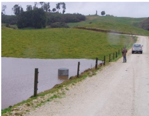
Figure 2.12: Retrofitted DB at Awahou site. Note: the raceway was already in place and riser was installed in 2012 to increase ponding time.
