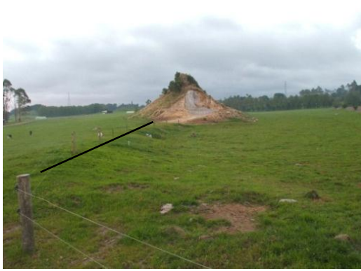
Figure 2.6: Hauraki DB (depicted by the black line), note the dry ponding area to the right, March 2012.
