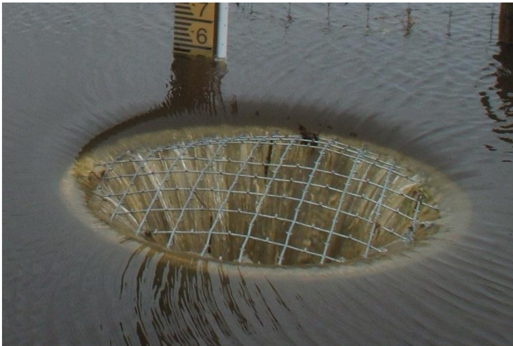
Figure 4.2: Water leaving the Waiteti DB over the riser in 2012. Note this water will have had a short residence time in the DB. Large volumes of water left via this riser in most storm events.
