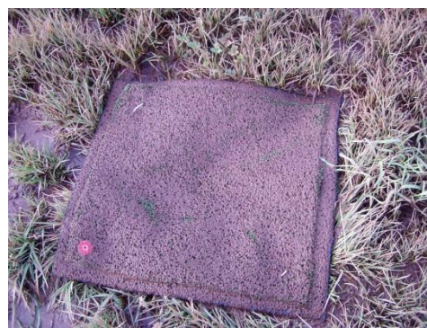
Figure 2.17: A synthetic turf mat after ponding at Awahou DB. Note this amount of sediment deposit is an extreme example.
