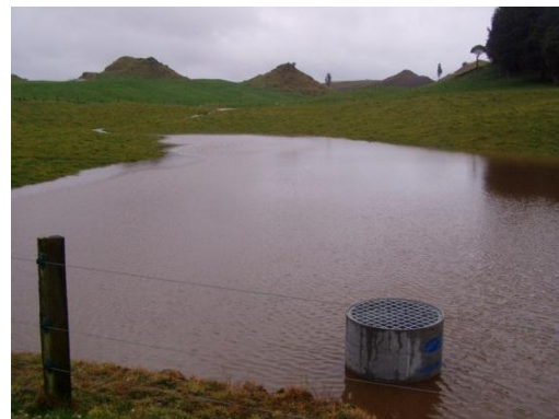
Figure 2.13: Ponded water at the Awahou DB, July, 2012.
