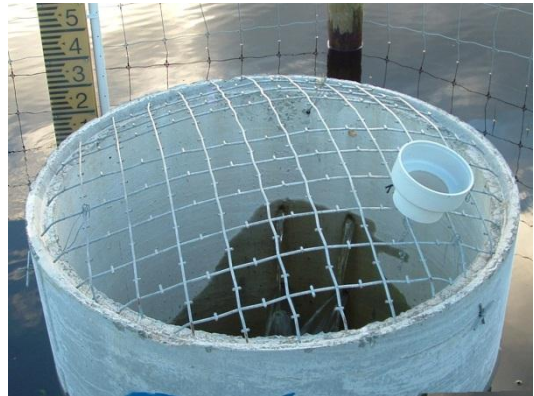
Figure 2.5: Water leaving the Waiteti DB via small holes in the riser, March 2012.
