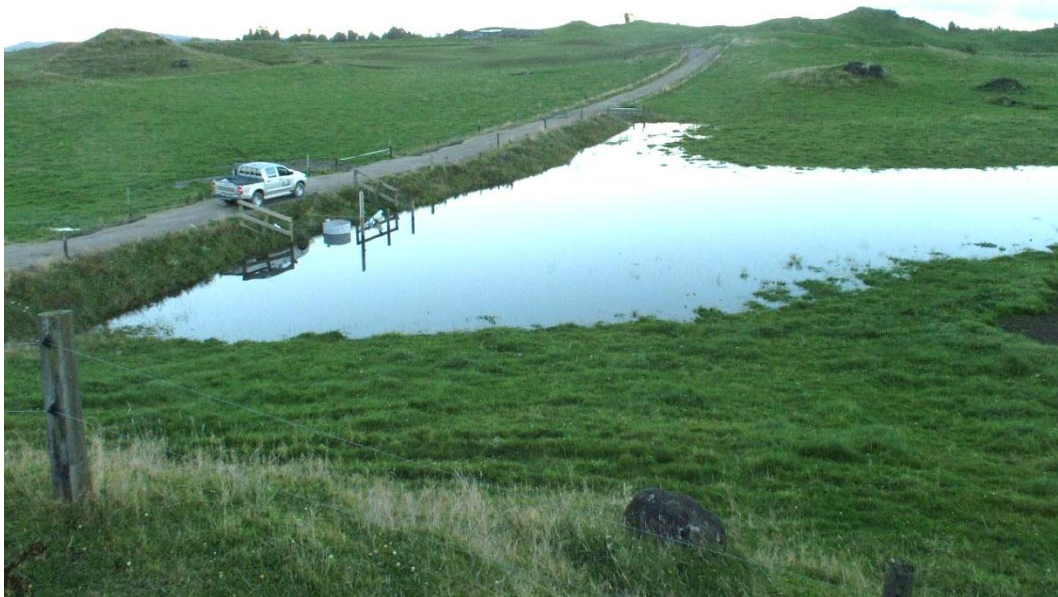
Figure 1.4: A typical detainment bund, designed to temporarily pond ephemeral stream water, Waiteti Stream catchment, Rotorua, March, 2012. This photograph has been taken after a runoff event and the pond is still draining.
