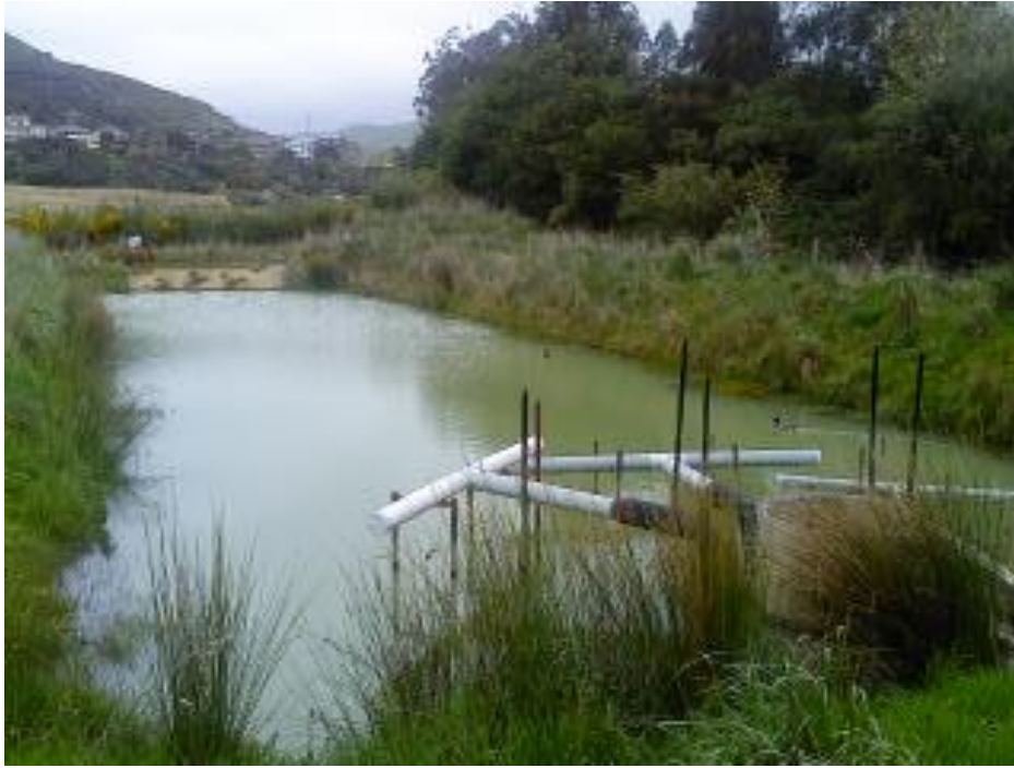
Figure 1.3: A Sediment Retention Pond used to attenuate sediment in runoff from construction sites. Note the suspended T-bar decant structure attached to a concrete riser allowing ‘dead’ storage of water. Courtesy of Goodman contracting, Wellington, 2012. Photo: Dylan Clarke, 5/10/2012).
