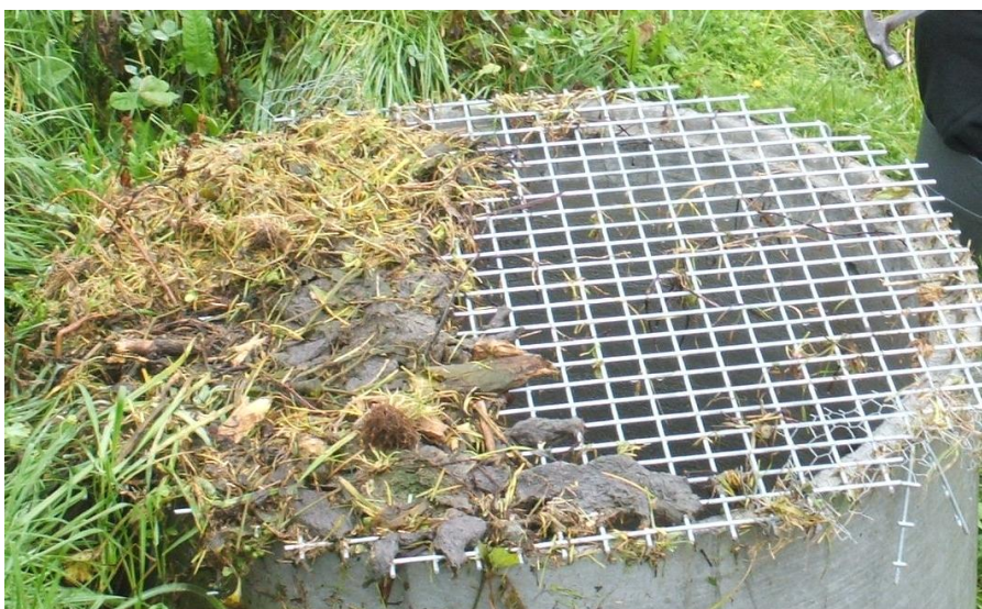
Figure 4.4 Agricultural debris deposited on a grate (20 mm spaces) on top of the riser at Hauraki DB after a ponding event in May, 2012. The debris is a potential hazard for outflow structures.
