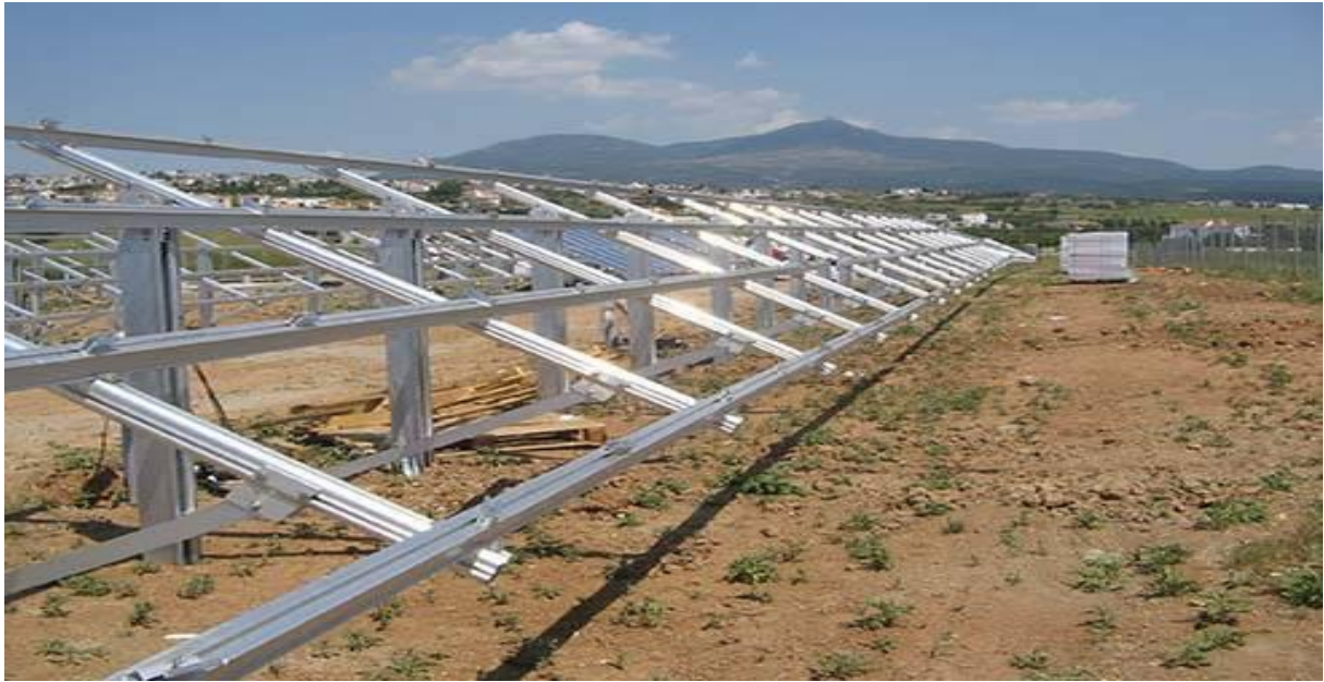
Fig: 4 Aluminium structure frame [8].
