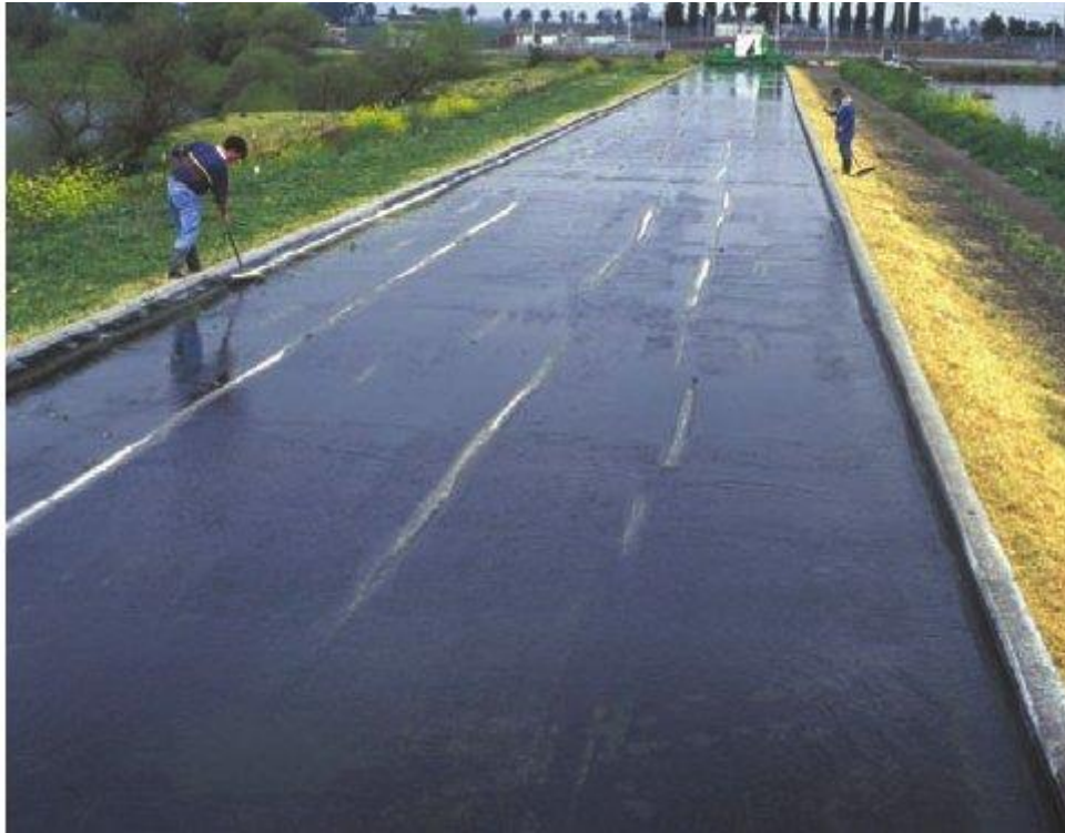
Figure 1.3: The large-scale ATS at Patterson, California, for secondary sewage treatment from 1994-1996 (after Adey et al., 2011)
