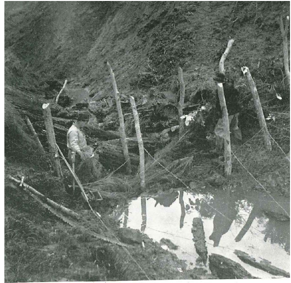
Fig. 11: Building No. 1 dam. A simple 2 row type. 20
