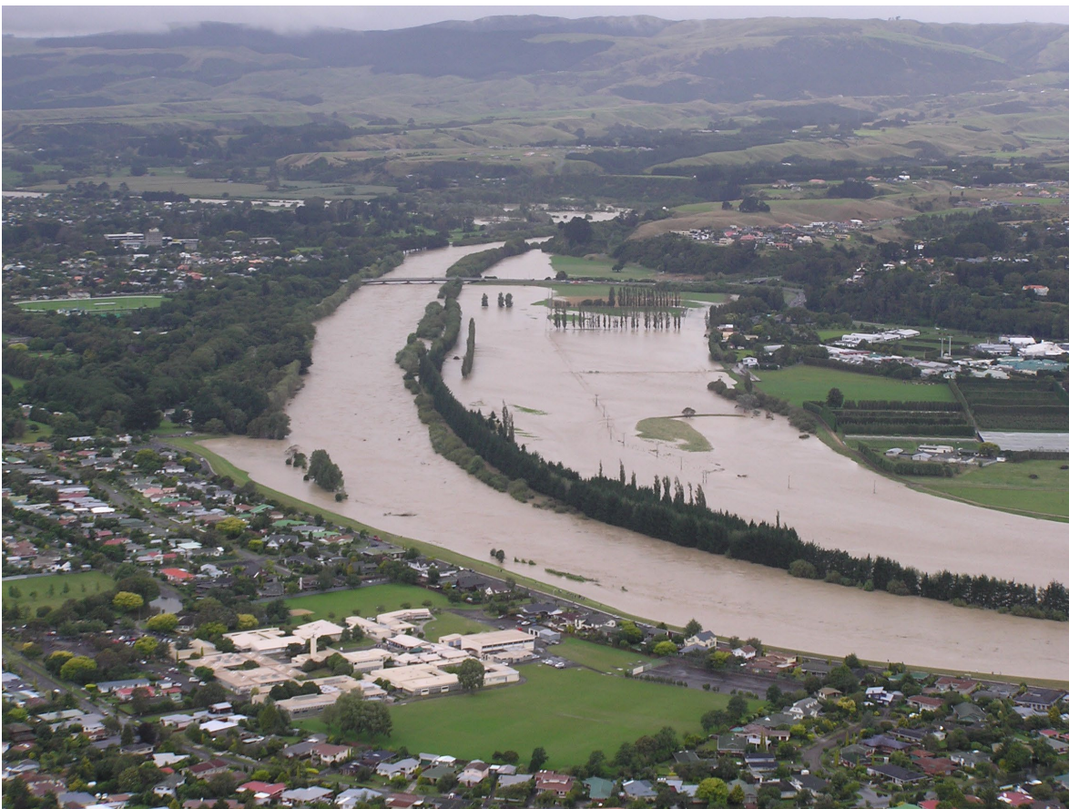
Fitzherbert Bridge, Palmerston North (February 2004).
