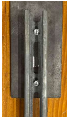
Figure 13 Double Screw connection
