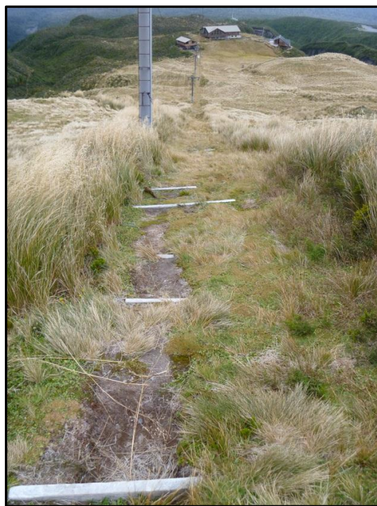
Figure 13: Retaining boards used by Manganui Ski Club to stabilise actively eroding areas on the lower ski field.
