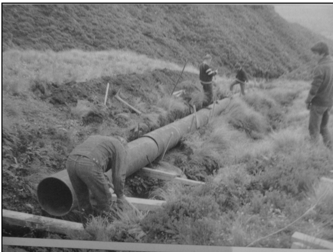
Figure 12: Photograph showing one of the large culverts being installed on the lower ski field in the 1980s (Stokes & Stokes 2001).
