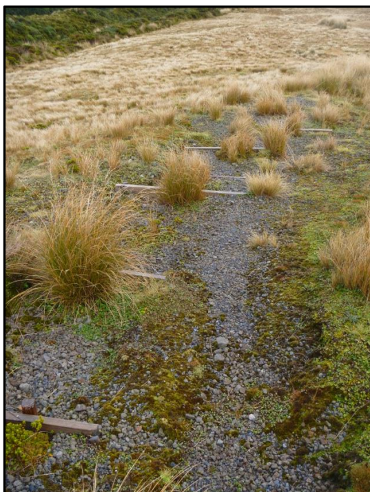
Figure 13: Retaining boards used by Manganui Ski Club to stabilise actively eroding areas on the lower ski field.
