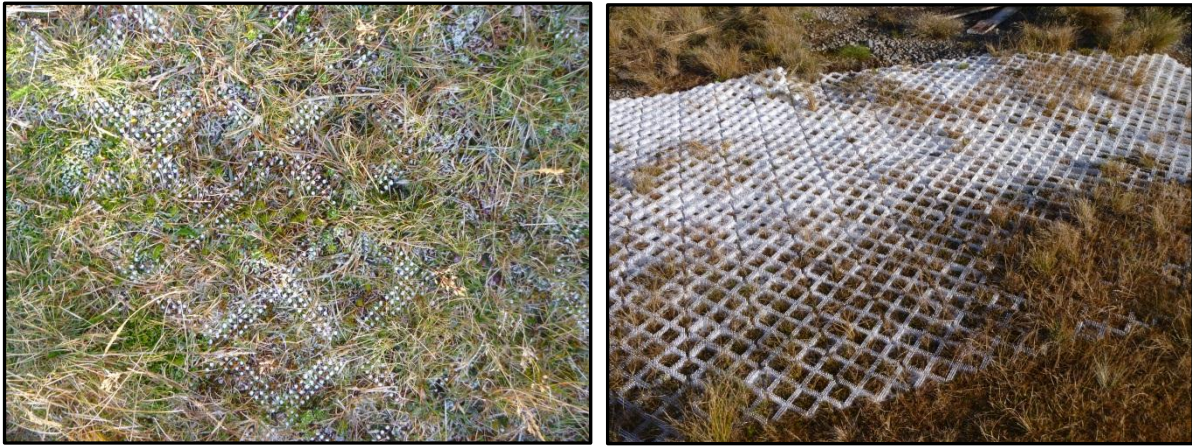
Figure 14: Snow mat tiles used under the T-bar tow line on the lower ski field.
