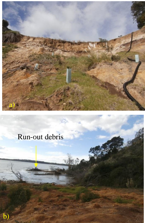
Figure 5.13: (a) Cliff scarp, (b) run off from landslip
