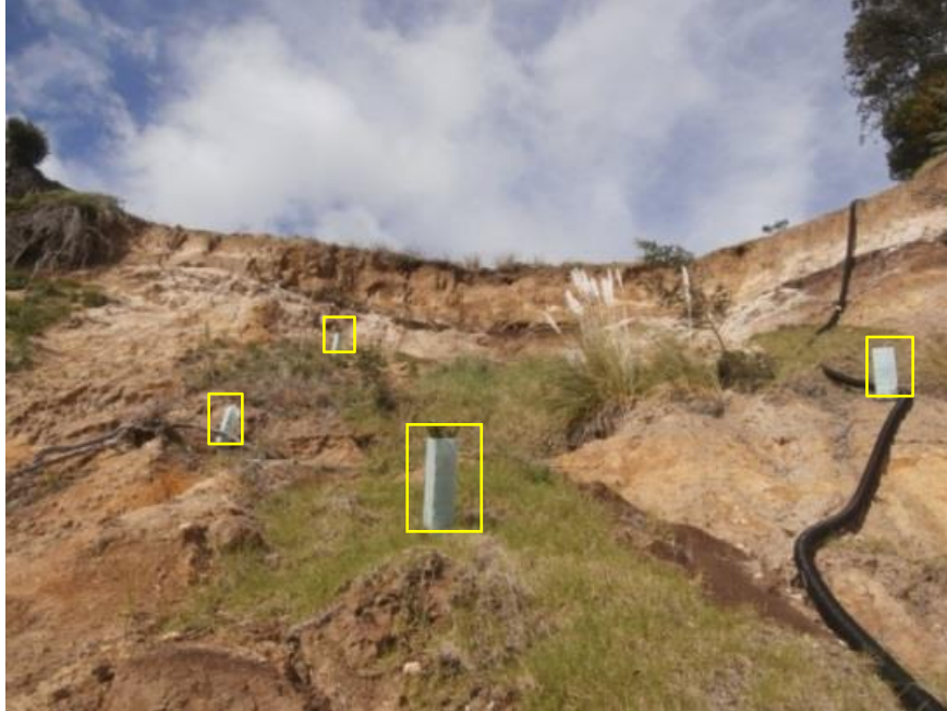
Figure 5.17: Poly pipes visible over the scarp and plants planted on the slopes of the scarp
