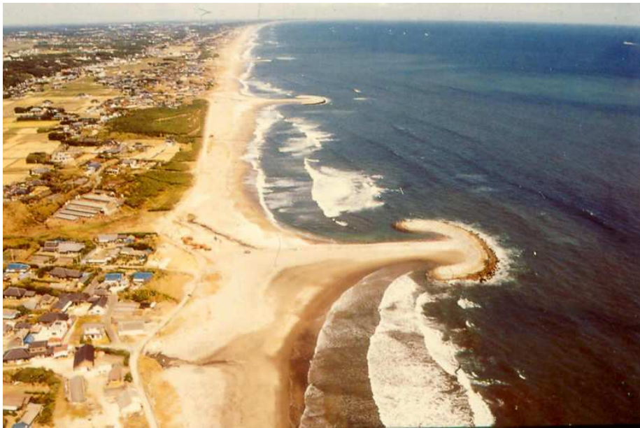
Figure 2.13: Artificial Headlands on the Ibaraki Coast Source: Japanese Coasts and Ports (1994) Committee on Coastal Engineering, Japan Society on Coastal Engineering, p.62.
