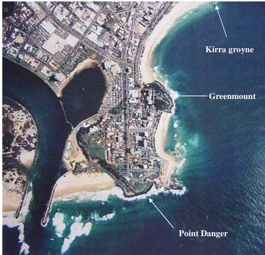
Figure 2.11: Aerial view of Point Danger to Kirra Point breakwater at the top of the picture, Gold Coast, Australia (Source: Gold Coast City Council, 23-4-96).
