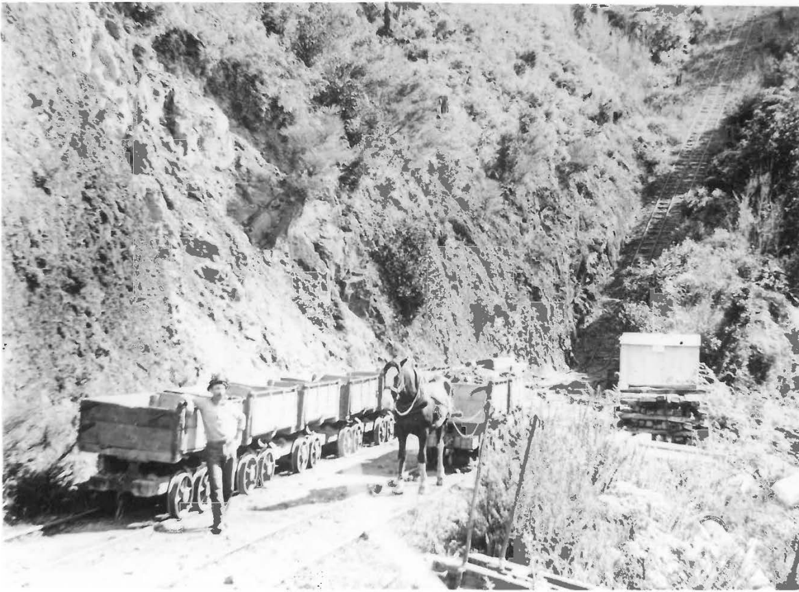
Figure 19: J.S. Hill, bottom of Butler's Spur Incline, with several wagons ready to be taken up and one to be carted downhill, n.d. [c. 1914], Eric Hill Collection.
