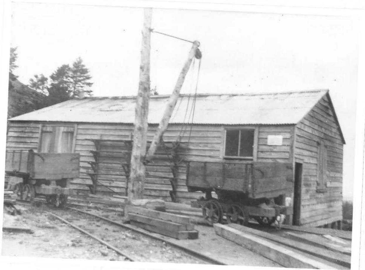
Figure 6: J.S. Hill, repair shop for tramway, at foot of Fern Spur, n.d. [c. 1914], Eric Hill Collection.
