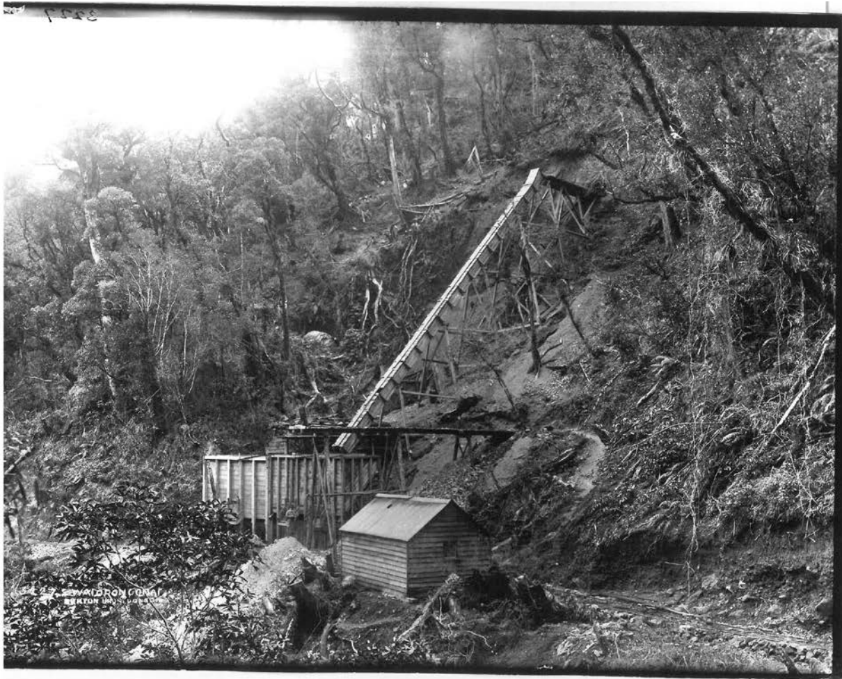
Figure 26: Burton Bros., chute and hopper beside tramway, 1884, C. 017248, Burton Brothers Collection, Museum of New Zealand Te Papa Tongarewa.
