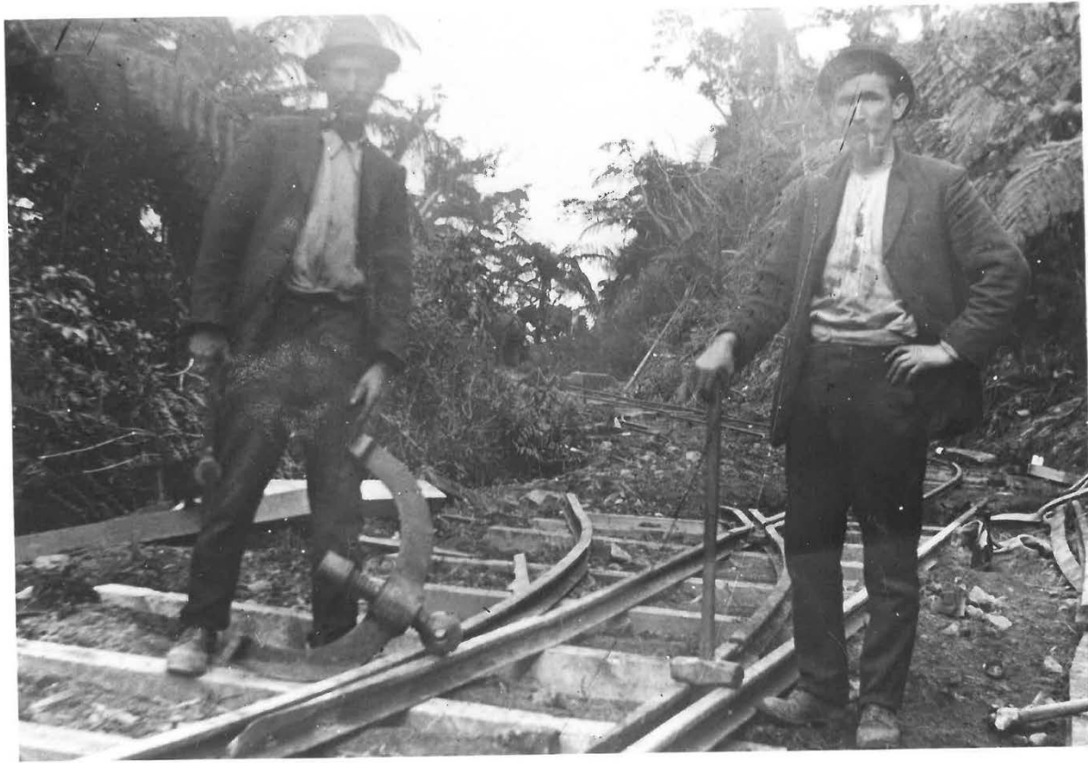
Figure 25: J.S. Hill, Men repairing tramway, n.d. [c. 1914], Eric Hill Collection.
