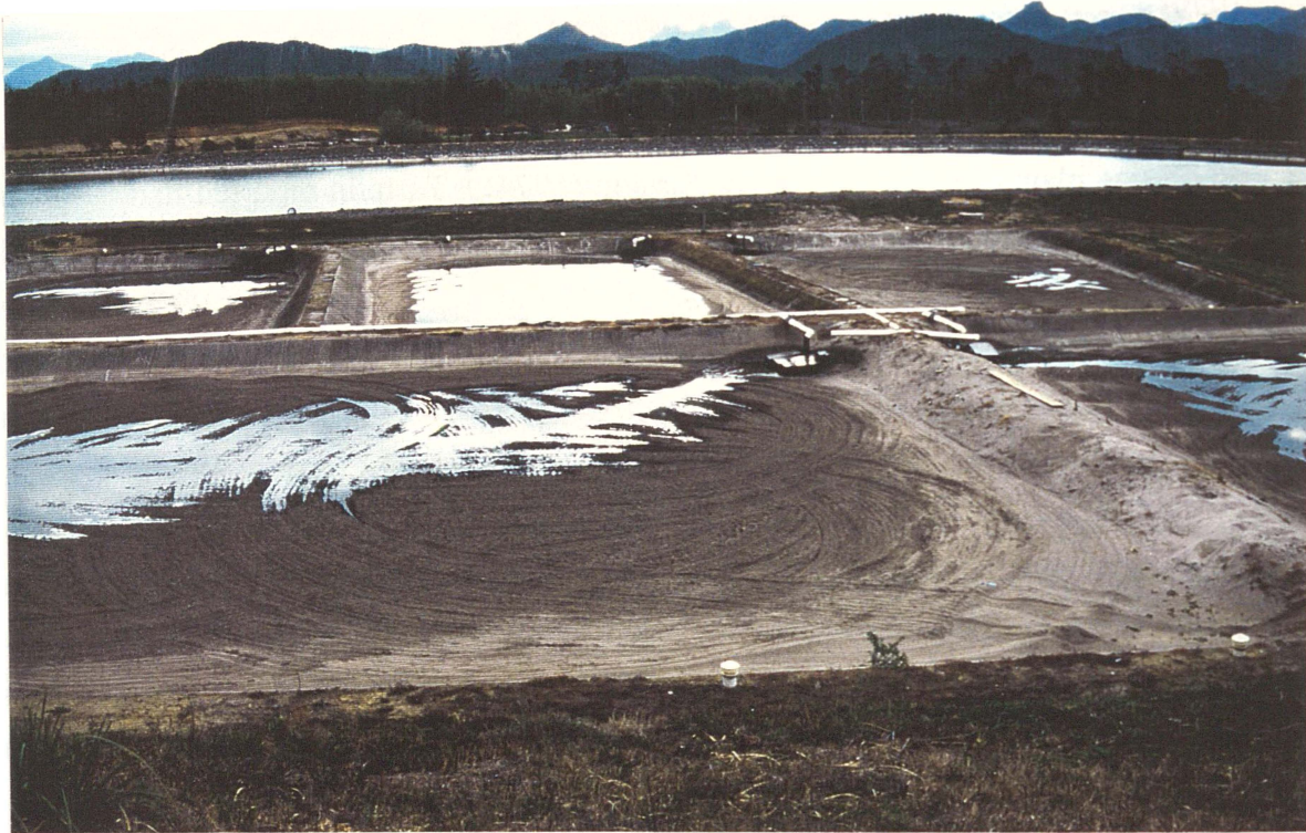
Figure 2.6 Rapid infiltration beds for sewage effluent treatment, Pauanui, New Zealand.
