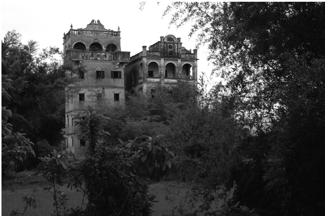
Plate 13: Soft foundations in low-lying land
