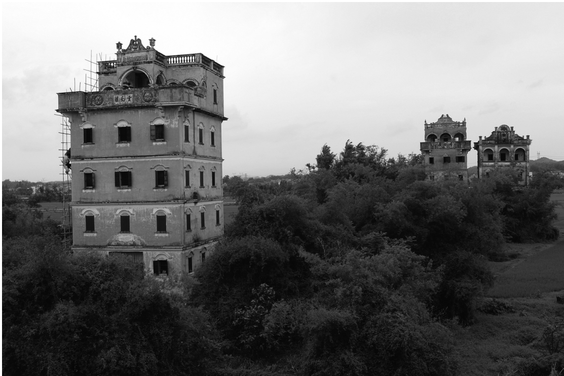
Plate 7: Diaolou undergoing restoration (notice the bamboo scaffolding)
