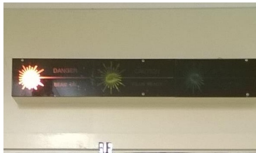
Figure 4.2.4: Laser status warning lights.
