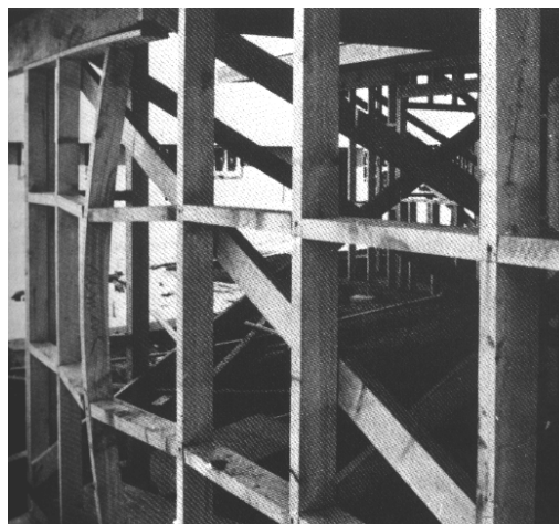
Figure 1.2 Warping of a stud in a fabricated wall due to compression wood (7) 1 .
