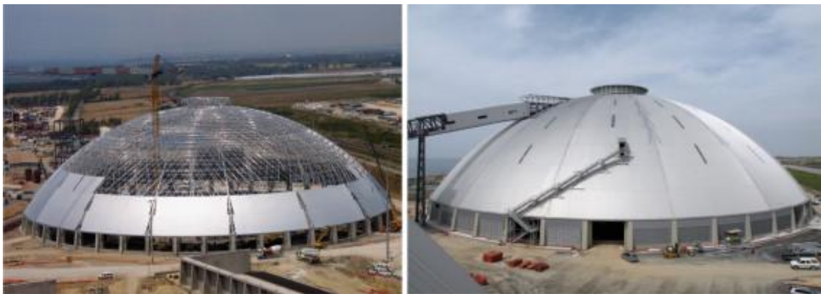
Fig. 2.9 shows two twin aluminium domes erected in the ENEL thermo-electrical power plant of Torrevaldaliga Nord (Civitavecchia, Italy) [34]
