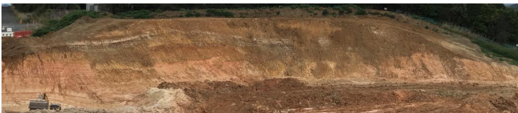
Figure 4.4 - Photograph of the NW face. Pictured to the far left (above digger) is the upper extent of the SW face.
