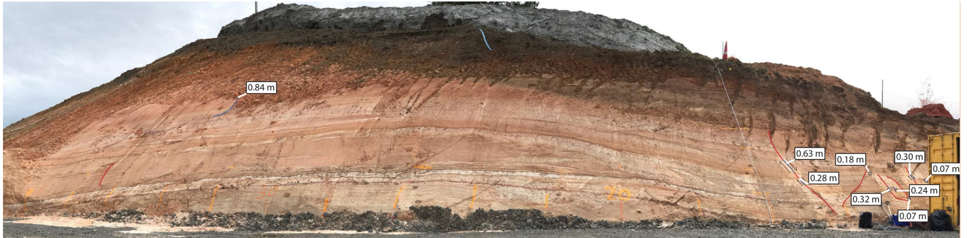
Figure 4.46 - Figure showing displacement within the SE face. As shown in this image, displacement was concentrated in the southernmost (right of image) portion of the SE face.
