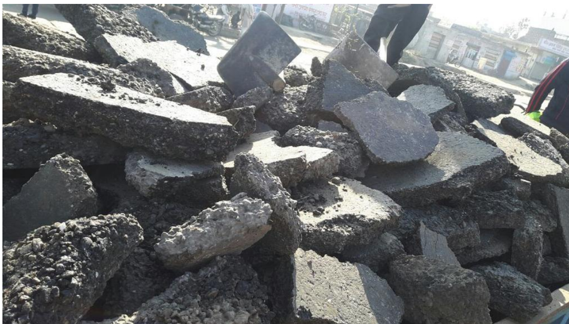
Figure 1. Chunks of RAP stockpiled.
