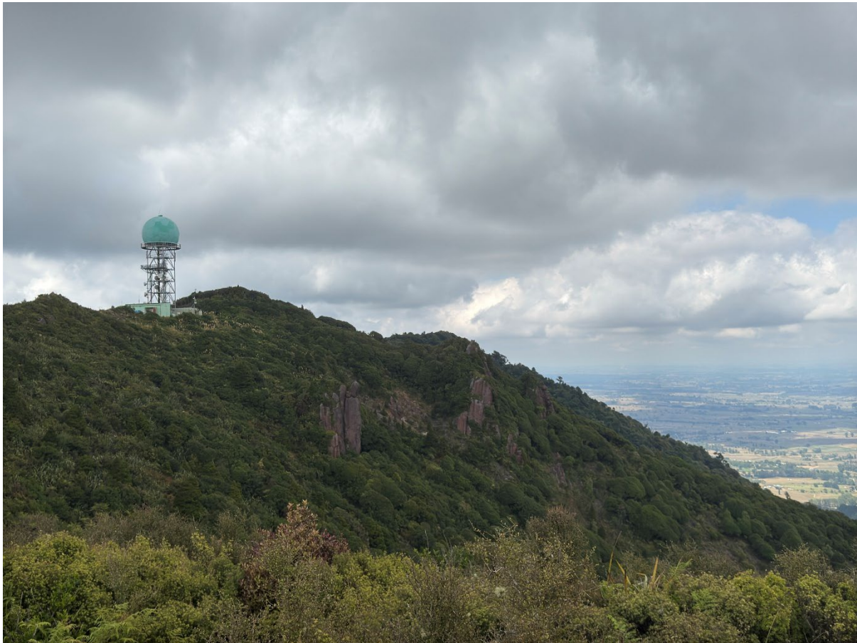
Figure 3.6: View looking south along the Te Weraiti ridge, showing the Civil Aviation Secondary Surveillance Radar installation with the Te Weraiti summit visible on the ridge behind it. Prominent rhyolite pinnacles are exposed on the western flank of the ridge below the radar installation. The near-vertical rocky outcrops represent exhumed dome core material, with the blocky, jointed rhyolite texture characteristic of viscous silicic lava emplacement. The steep western margin dropping toward the Waikato Basin is visible to the right, illustrating the pronounced topographic relief and asymmetric morphology of Te Weraiti consistent with fault-influenced emplacement along the Kaimai Range front. The dense native vegetation cover across the dome flanks is indicative of the limited rock exposure encountered during field investigation.
