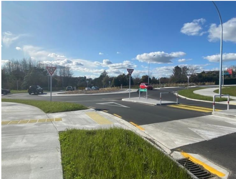
Figure 14. Napier/Kiddle/Arrowsmith roundabout with RSPs in Taupo, NZ.
