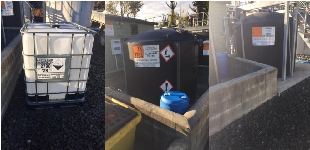
Figure 12. Photos showing the acetate, alum, and soda ash which was added to the treatment plant at different times throughout the year.
