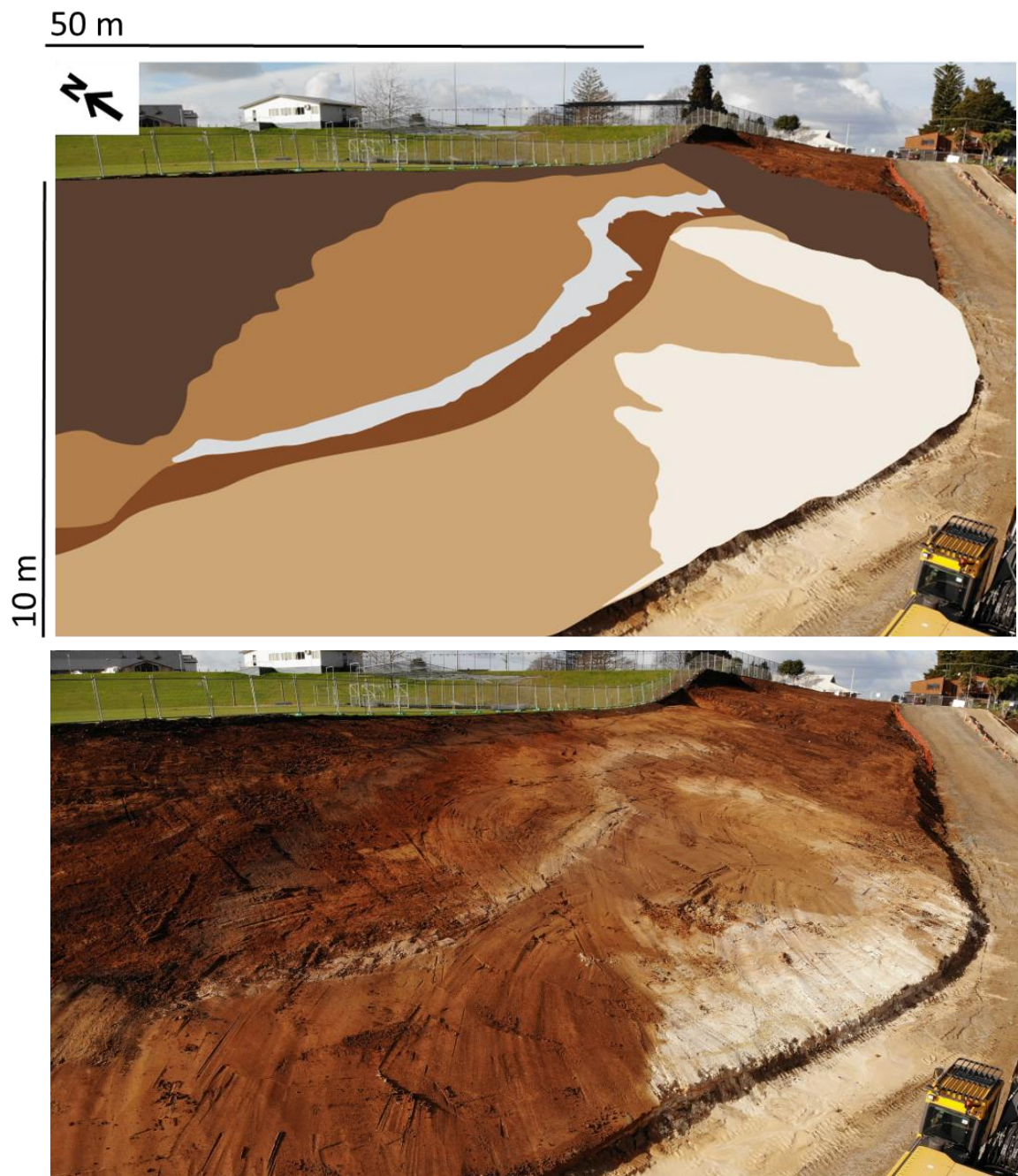
Figure 4.5 Inkscape annotation of cutting presenting stratigraphic relationships at 59 Hillcrest Road, Hamilton. Facing east-northeast.
