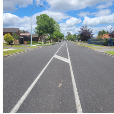
(b) LTS2. Speeds and traffic volumes are low, and there is only one lane per direction. Most people would feel comfortable biking on a road like this. (Ashurst Avenue – Kirikiriroa Hamilton)
