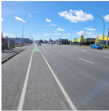
(c) LTS3. Dedicated bicycle infrastructure is unprotected and beside high speed, multi-lane traffic. Only a few people would feel comfortable biking on a road like this. (Te Rapa Straight – Kirikiriroa Hamilton).
