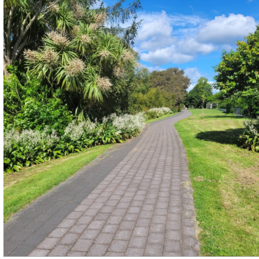
(a) LTS1. Completely separate bicycle infrastructure. All cyclists, including children, would feel comfortable biking on a path like this. (Te Awa River Path – Kirikiriroa Hamilton)
