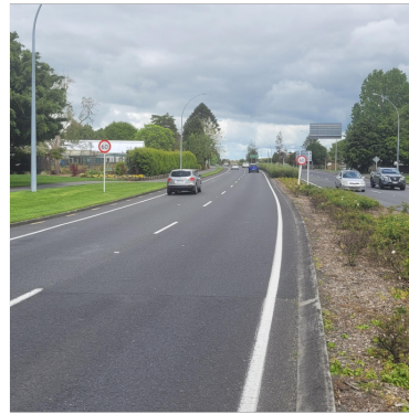
(d) LTS4. No dedicated bicycle infrastructure, high speeds, and multiple through lanes per direction. Most people would avoid biking on this road. (Cobham Drive – Kirikiriroa Hamilton)
