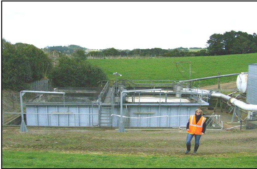
**Figure 7.3** A site wastewater sump at the Fonterra Kauri dairy factory, Northland in New Zealand.
