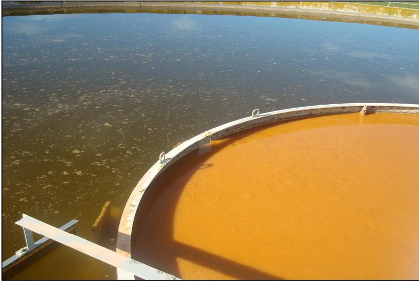
**Figure 4.5** Clarifiers where the floc is separated from the water by gravity at the Waitoa dairy wastewater treatment plant.
