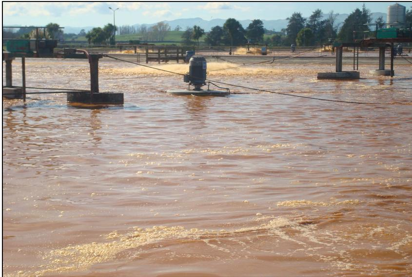
**Figure 4.4** An extended aeration sludge wastewater treatment pond, where the activated sludge uses dairy wastewater as a food source and consumes oxygen to satisfy the micro-organisms.
