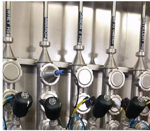
Figure 3-6. YSI Professional Plus (Pro Plus) Multiparameter Instrument screwed directly into the Awaroa effluent line.
