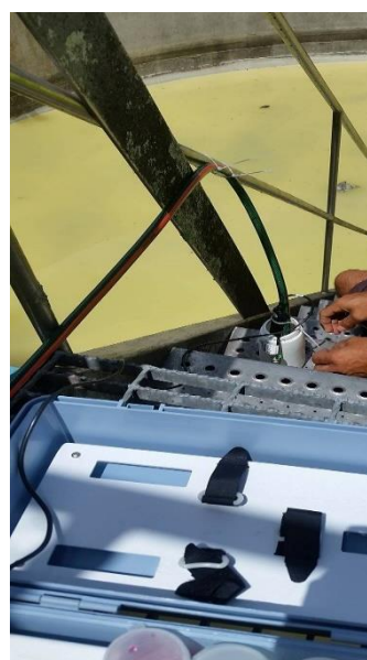
Figure 3-11. Hose running into holding tank.
