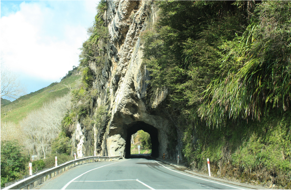
Frontispiece: Awakino Tunnel at the northern end of Awakino Gorge is cut through steeply dipping Orahari Limestone (late Oligocene, Duntroonian, Ld) of the Te Kuiti Group (see Stop 10).
