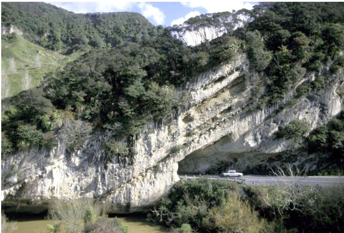
Fig. 21. Orahiri Limestone at Awakino Tunnel (see also Frontispiece photo). The mainly recessive beds in the cliff above the tunnel entrance are a succession of redeposited beds containing lithoclasts (Limestone-in-limestone Beds of Nelson 1978).
