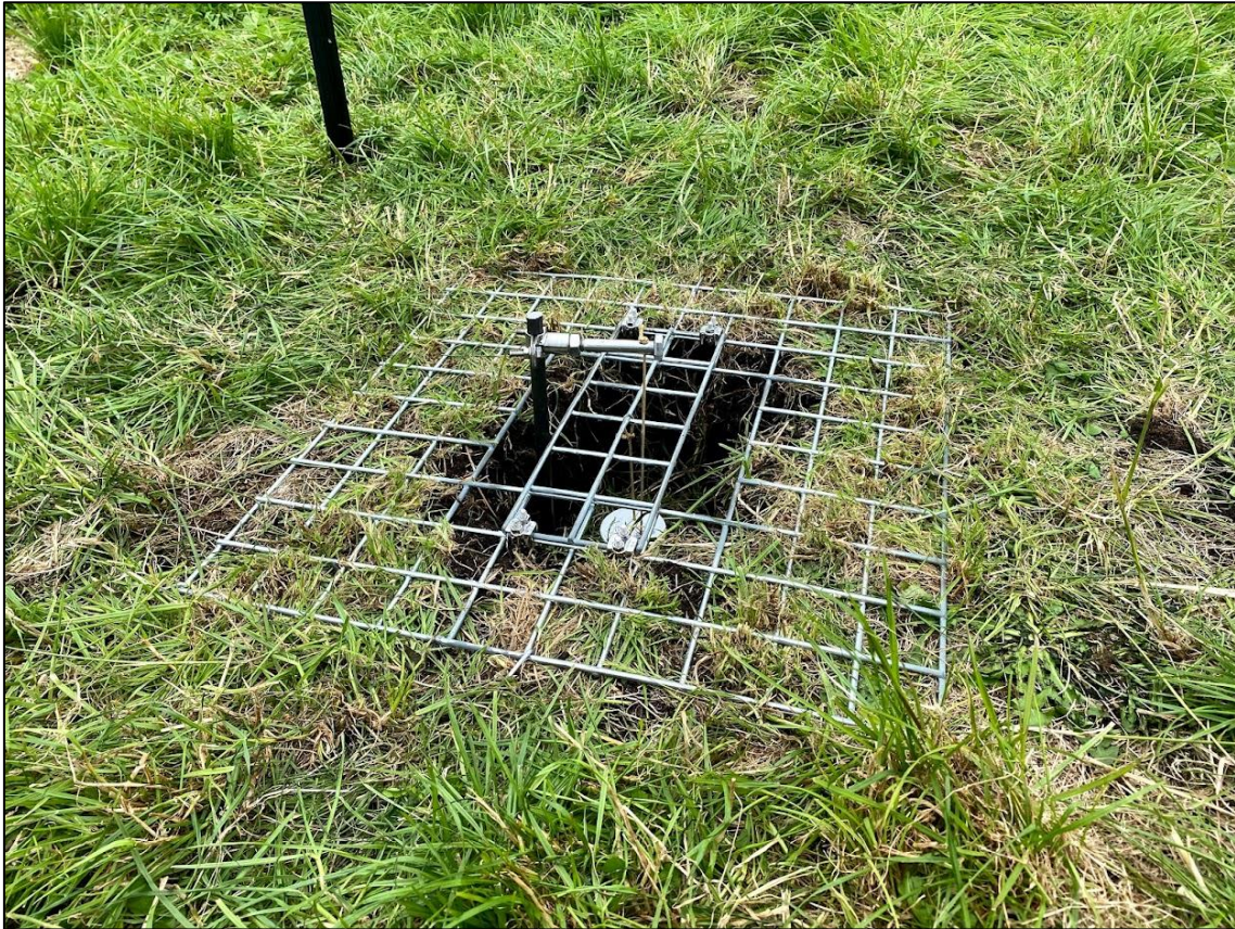
Figure 3.8 Photograph of aboveground hardware at the Moa_Dairy PSO site, showing the steel benchmark rod, horizontal bolt with AWL probe Kevlar cord attachment, steel mesh with RWL probe attachment and dipwell cap through which Kevlar lines ran. (Photo credit: David Campbell, 2021)
