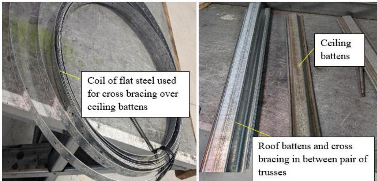
Figure 3-14: Coil of flat steel used for bracing, roof batten and ceiling batten
