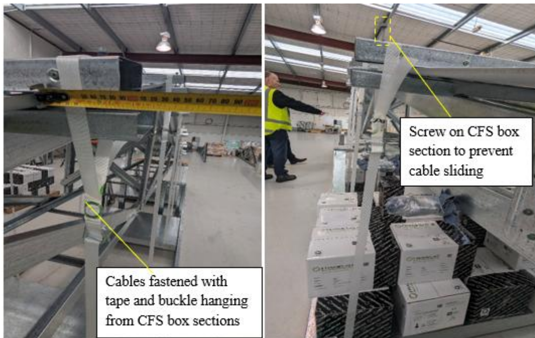
Figure 3-25: Loaded pallets hanging from CFS Box Sections
