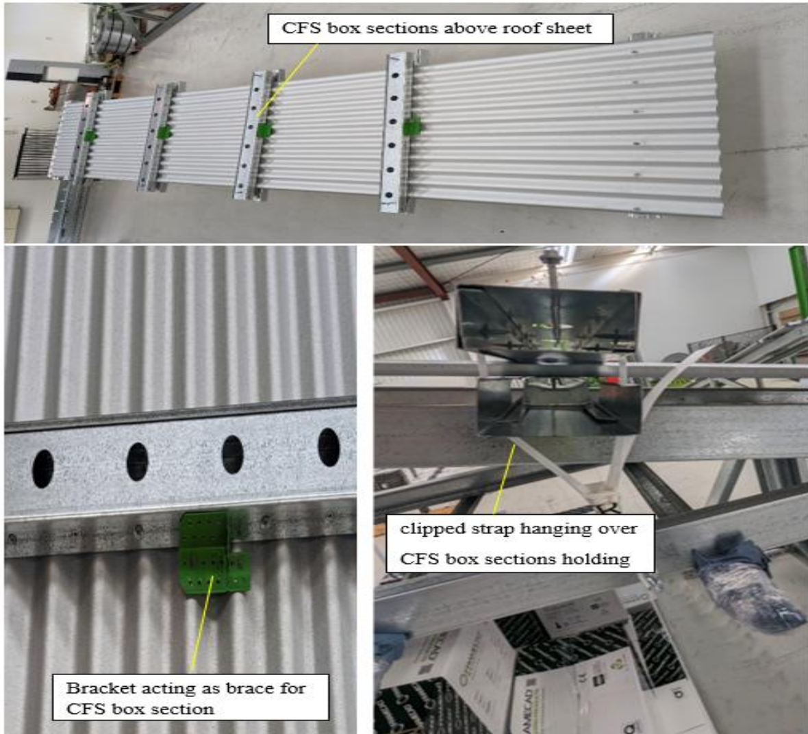
Figure 3-22: CFS Steel Box Sections on Roof Sheets
