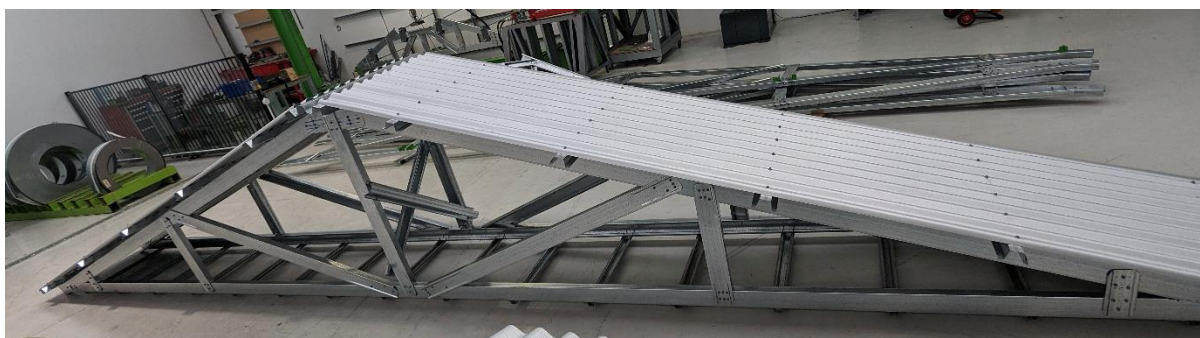
Figure 3-11: Roof Truss Assembly Set up
