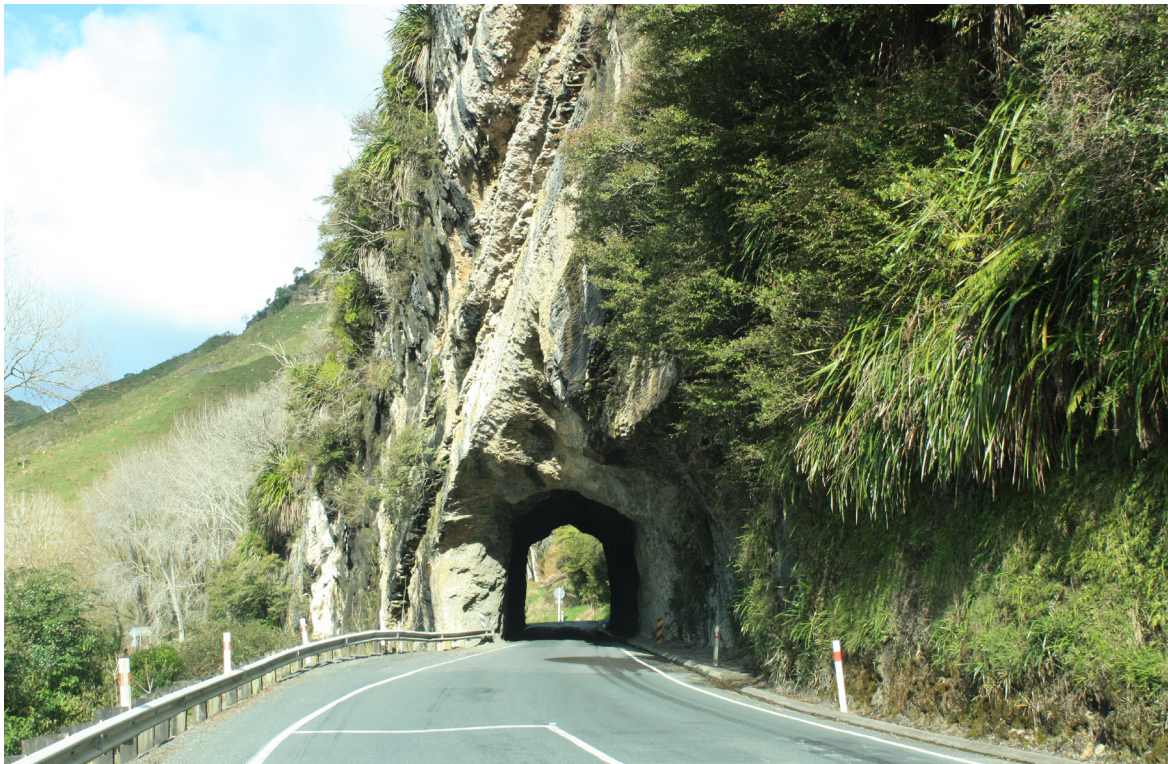
Frontispiece B. Awakino Tunnel at the northern end of Awakino Gorge is cut through steeply dipping Orahiri Limestone (late Oligocene, Duntroonian, Ld) of the Te Kuiti Group (Stop 10, R17/615854).
