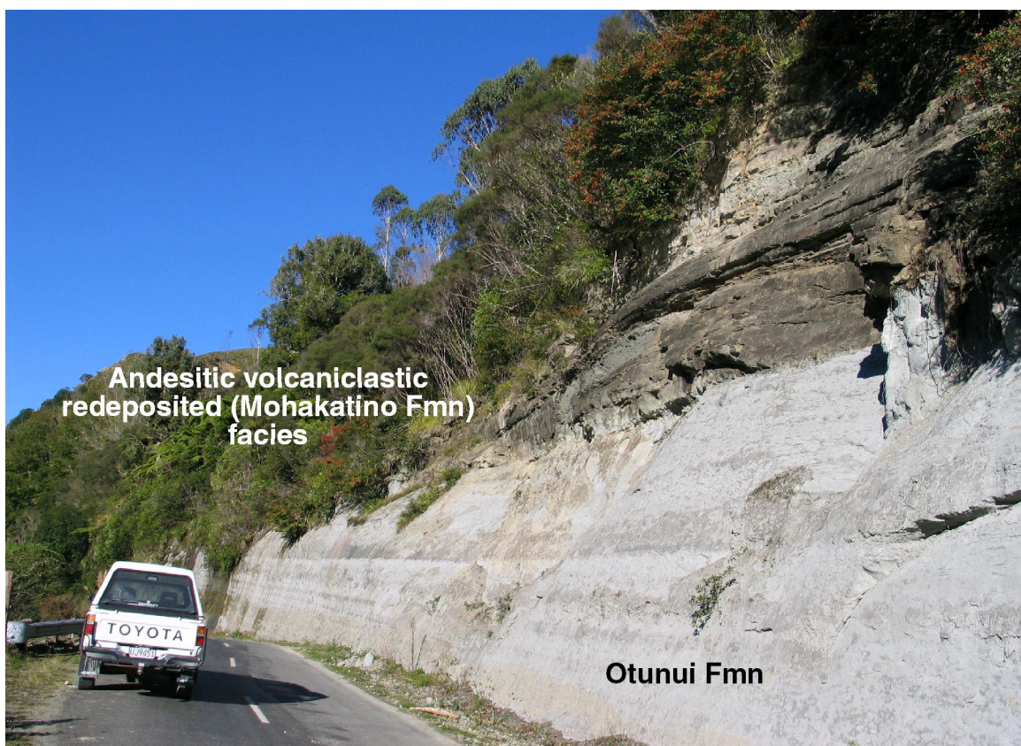
Fig. 36. Otunui Formation at Okau Road that includes a thin interbedded unit of volcanoclastic Mohakatino Formation.
