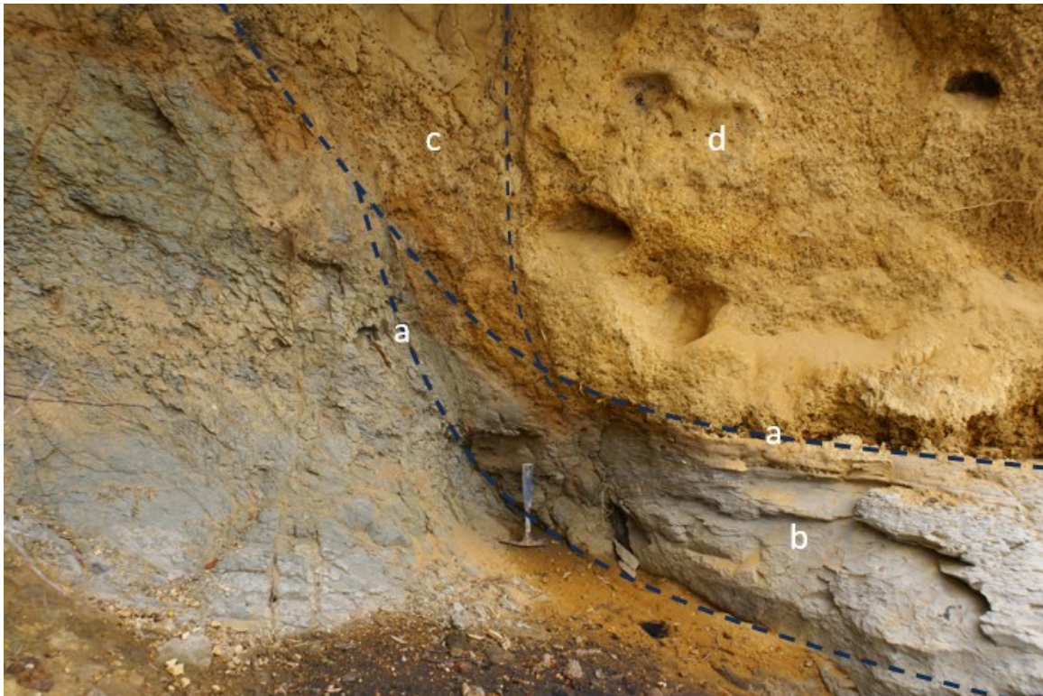
Figure 3.7: Fault planes (a) in Whaingaroa Siltstone (b). Shearing \leq 26.5 ka Kaihu Group pumiceous sand (c; d). Vertical displacement is > 1 m. Horongarara Peninsula, Raglan Harbour.
